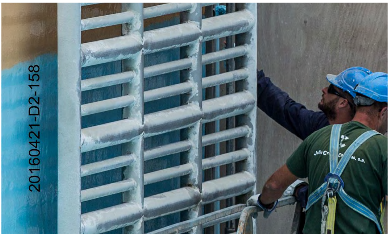
Figure 16. The medical tank segregation gates are constructed with heavy pipe-metal and are at both the west and east ends. A sense of scale is perceived when comparing the main cross pipes to the similar thickness of the man’s arm (also see Figure 14). Based on the known dimensions of the medical tank, the gates are more than 4m (13.12ft) high and approx. 3m (9.84ft) wide.
